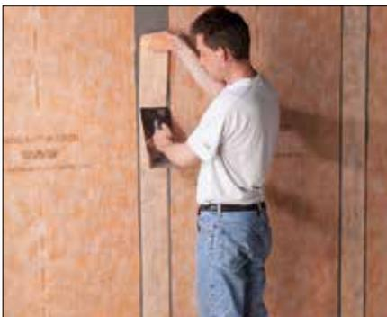
**4** The prefabricated Schlüter-KERDI parts can be used for internal and external corners, while the pipe collars Schlüter-KERDI-KM or Schlüter-KERDI-MV are suitable for pipe penetrations.
