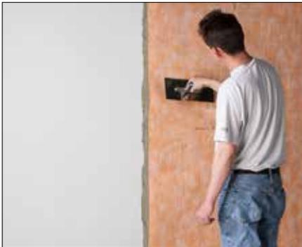
**3** Joints can be constructed by overlapping the edges of the Schlüter-KERDI 5 cm or by abutting the edges and covering the joint with 12.5 cm wide Schlüter-KERDI-KEBA band. Use the sealing adhesive Schlüter-KERDI-COLL-L to seal the abutting seams and overlaps.
