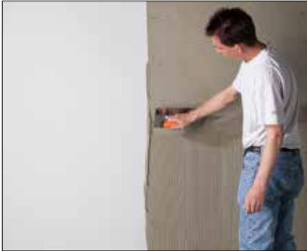
**1** The substrate must be clean, even, and load bearing. Cut Schlüter-KERDI to size prior to application, using scissors or a utility knife.
