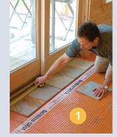
1 After tiles are dry-fit in front of the door, measuring the width of the room determines whether the layout should be centered on a tile or on a grout joint for the best use of materials.
