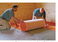
**One course at a time.** Spread only enough mortar for one course of membrane, then roll out the precut pieces.
