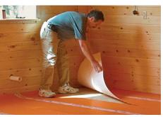
**Test-fit first.** Cut membrane to fit the floor with scissors or a utility knife. Cover the subfloor completely.
