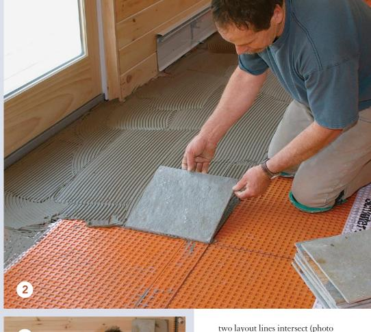
two layout lines intersect (photo top right). As I work down the floor, I apply thinset to an area in which I can set tile within about 15 minutes, usually about 30 sq. ft. at a time. For each set of courses, I install the first tile at the intersection of the layout lines. As each tile goes in, I apply a little downward pressure and slide the tile into place, which helps to lock the tile into the layer of thinset.
