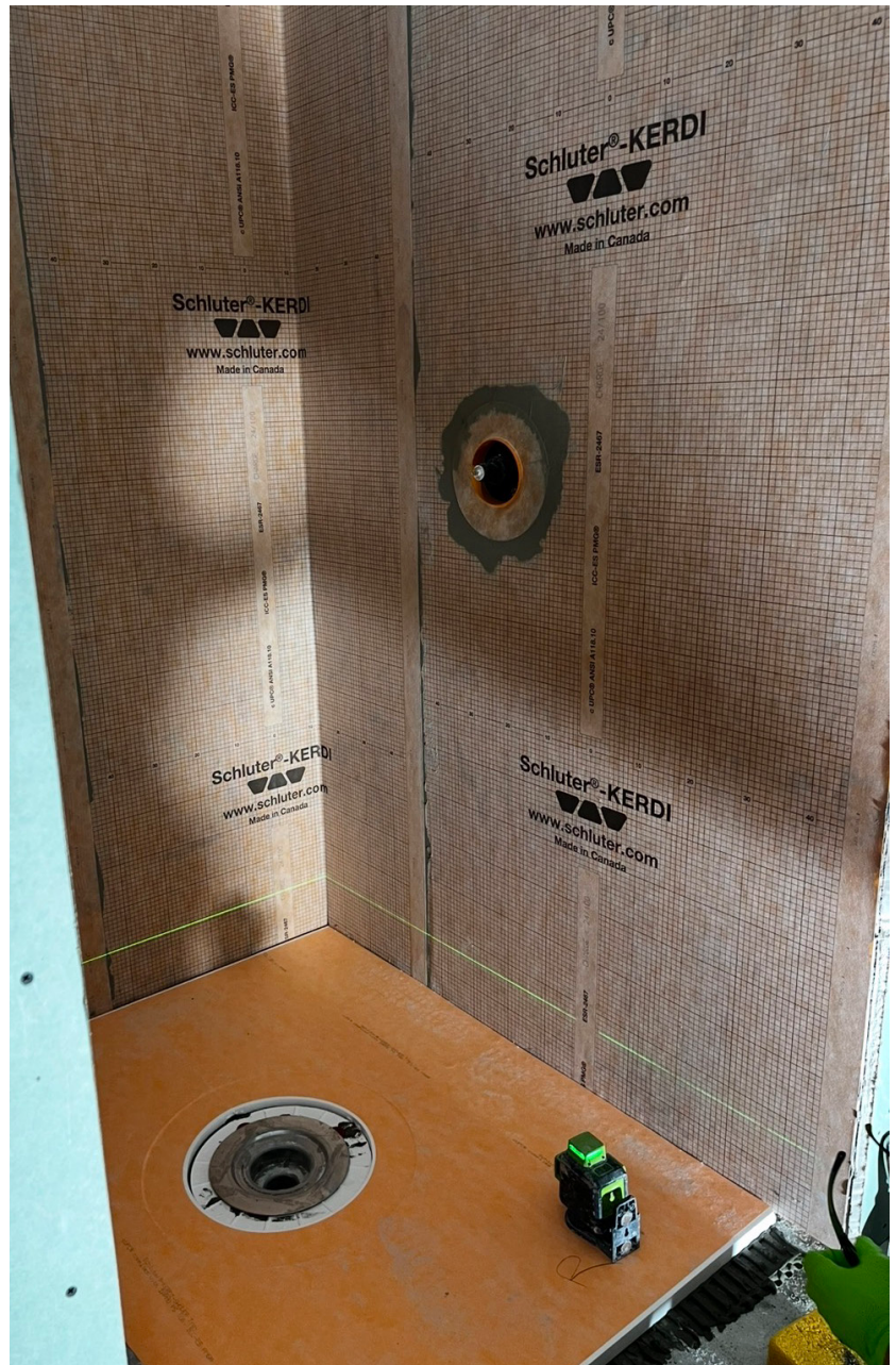
In-progress installation showing Schluter®-KERDI waterproofing membrane and prefabricated shower tray.
