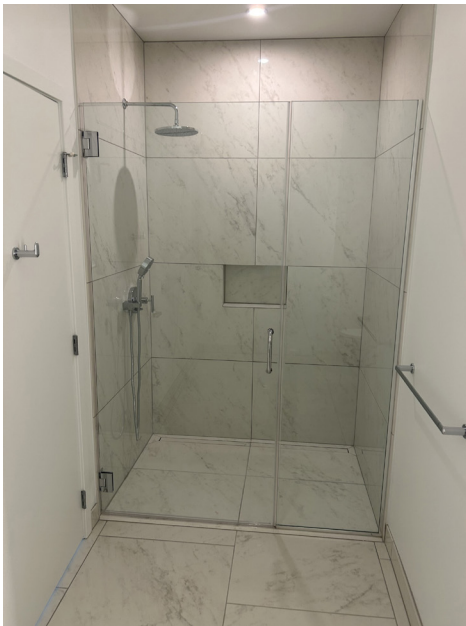
Finished shower with large-format porcelain tile and Schluter®-KERDI-LINE linear drain for curbless entry.
