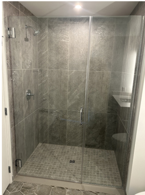
Completed unit shower with dark stone tile, point drain, and consistent grout alignment.
