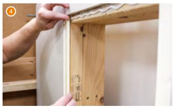
Using the supplied tube of KERDI-FIX, glue the spacers to the studwork frame.
