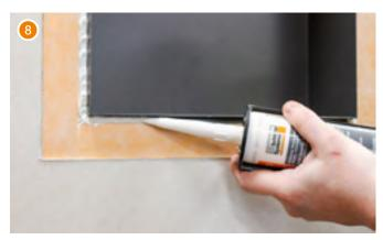
Use KERDI-FIX to completely fill the joint between the niche body and the niche frame.
