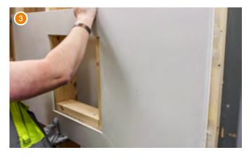
Fix the plasterboard with the hole cut in it (step 2) to the studwork so the hole and studwork frame align
