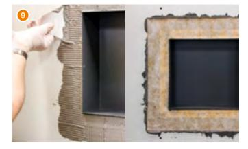
Using KERDI-COLL-L-185 adhere the KERDI-collar to the niche frame and surrounding plasterboard, creating a waterproof seal
