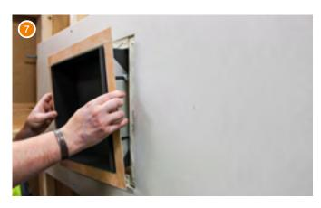
Slot the niche into the opening, gently pushing the frame on to the KERDI-FIX on the surface of the spacers  $\,$
