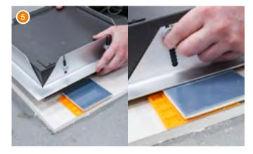
Using the piece of plasterboard cut out in step 2 and the wall tile that will be used (plus a small piece of DITRA-PS to mimic a bed of tile adhesive) as a guide, use the adjustable nuts on the niche body to slide it backwards or forwards until it is set to the required depth - either flush with the surface of the tiled wall or protruding out from the tiled wall - and tighten the nuts
