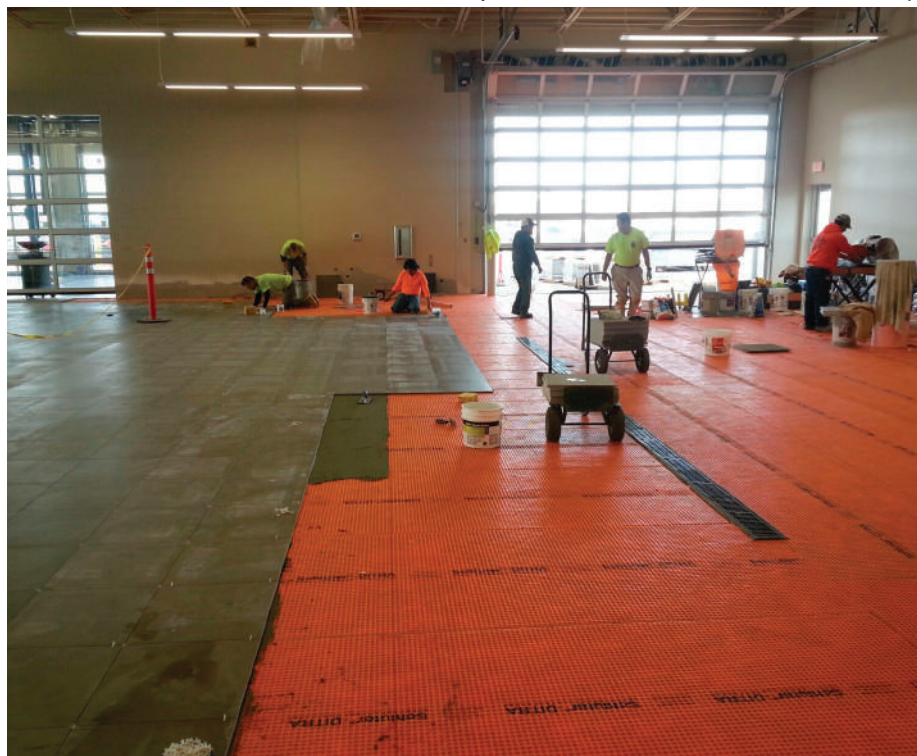
The floors would be subject to frequent and heavy vehicular traffic so Schluter-DITRA was used in the entire area to provide the necessary load support and uncoupling. Photo credit: Mesa Tile and Stone
