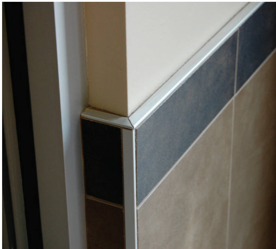
The top of the tile base and wainscot were trimmed with a flat profile with an aluminum anodized finish. Photo credit: Mesa Tile and Stone.
