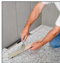
re 5. Apply cementitious tile adhesive to covering support
