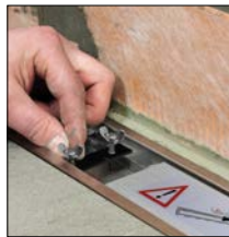
re 2. Use height adjustment aid to adapt the frame ...
