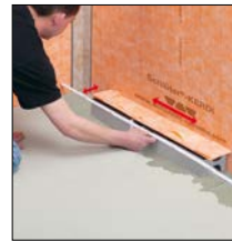
re 4. Align channel support
