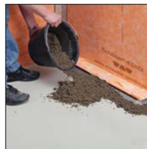
re 5. Apply screed
