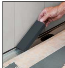
re 2. Place spacers in the channel body
