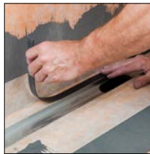
re 1. For wall installation: adhere cover strips facing the wall
