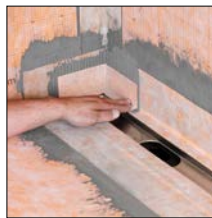
re 3. Retrofit KERECK internal corner
