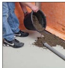
re 6. Apply sloped screed
