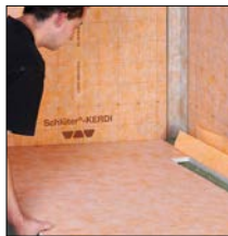
re 3. Push sloped tray under the edge of the channel body
