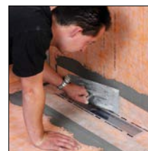
re 4. KERDI collar adhere with KERDI-COLL-L
