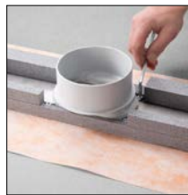
re 3. Screw adapter back on
