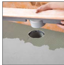
re 4. Place channel body including channel support
