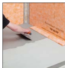
re 7. Apply cementitious tile adhesive
