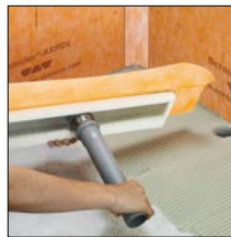
re 2. Insert drain pipe
