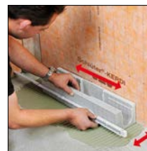
re 1. Align channel support
