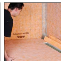
re 3. Push sloped tray under the edge of the channel body
