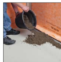
re 3. Apply levelling screed
