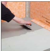
re 6. Apply thin-bed mortar
