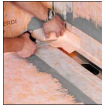
re 2. Adhere the KERDI collar/cut the KERECK internal corner to size
