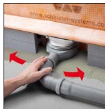
re 5. Align drainage pipe
