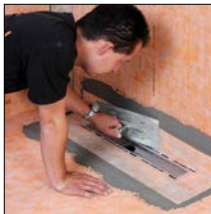
re 4. KERDI collar adhere with KERDI-COLL-L
