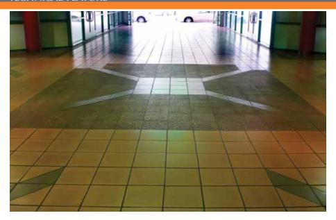
This tiled floor on the ground-level public/retail areas of Phoenix Plaza in Oakland, Calif., was installed in 1989. It was set over DITRA uncoupling membrane, installed on post-tensioned concrete over a parking garage. It has endured frequent use – including the 7.1 Loma Prieta earthquake – and is still in excellent condition today.
