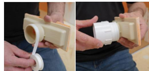
**3** Attach the foam supports to the flange using Schluter®-KERDI-FIX, Schluter SET®, ALL-SET®, FAST-SET®, or unmodified thin-set mortar. **Note:** The foam supports only fit one way to align with the off-center flange outlet.
