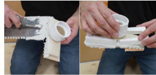
**Plumbing Access:** When there is no access to the plumbing from below, the flange must be set and connected to the waste line simultaneously according to Step 7. When there is access to the plumbing from below and the waste pipe can be connected after installing KERDI-LINE-VARIO, you may skip Step 7.
