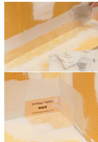
**Note:** A flood test is strongly recommended before setting tile to verify a successful installation. Wait a minimum of 24 hours after the membrane installation is complete to allow for final set of thin-set mortar and ensure waterproof performance at seams and corners. Refer to local plumbing codes for any specific requirements in your area.
