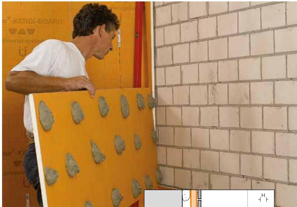
Schlüter-KERDI-BOARD can be fully adhered in wall areas or alternatively attached with dabs of adhesive. If necessary, the material may be secured with additional wall anchors. In the case of stud frames made of wood or metal, Schlüter-KERDI-BOARD is attached with screws from the matching hardware system.
