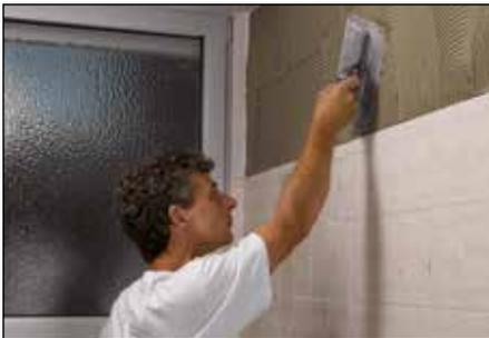
Schlüter-KERDI-BOARD is made from an extruded XPS hard foam, with a cement-free reinforcement layer laminated onto both sides, together with an anchoring fleece webbing. The grid imprint on one side provides ideal guidance for cutting the boards to size.
